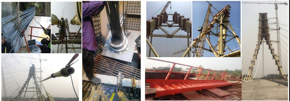
Fig.20 Cable installation, tensioning and Pylon access system during construction
