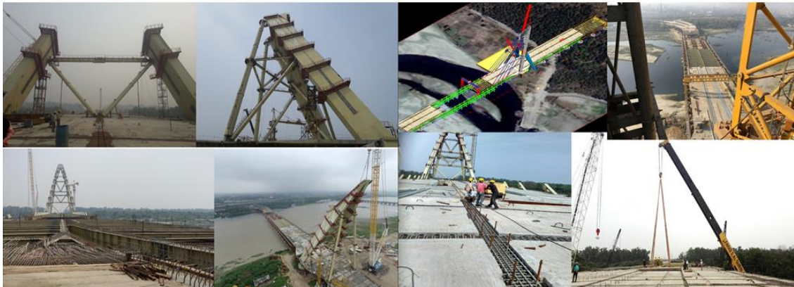
Fig.13. Temporary supports for erection & Deck erection by Goliath gantry & crane
