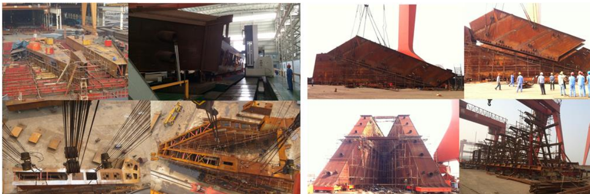
Fig.11. Fabrication, machining and trial assembly of pylon kink and L6 –L10 and M0, M1and M2, and pylon head
