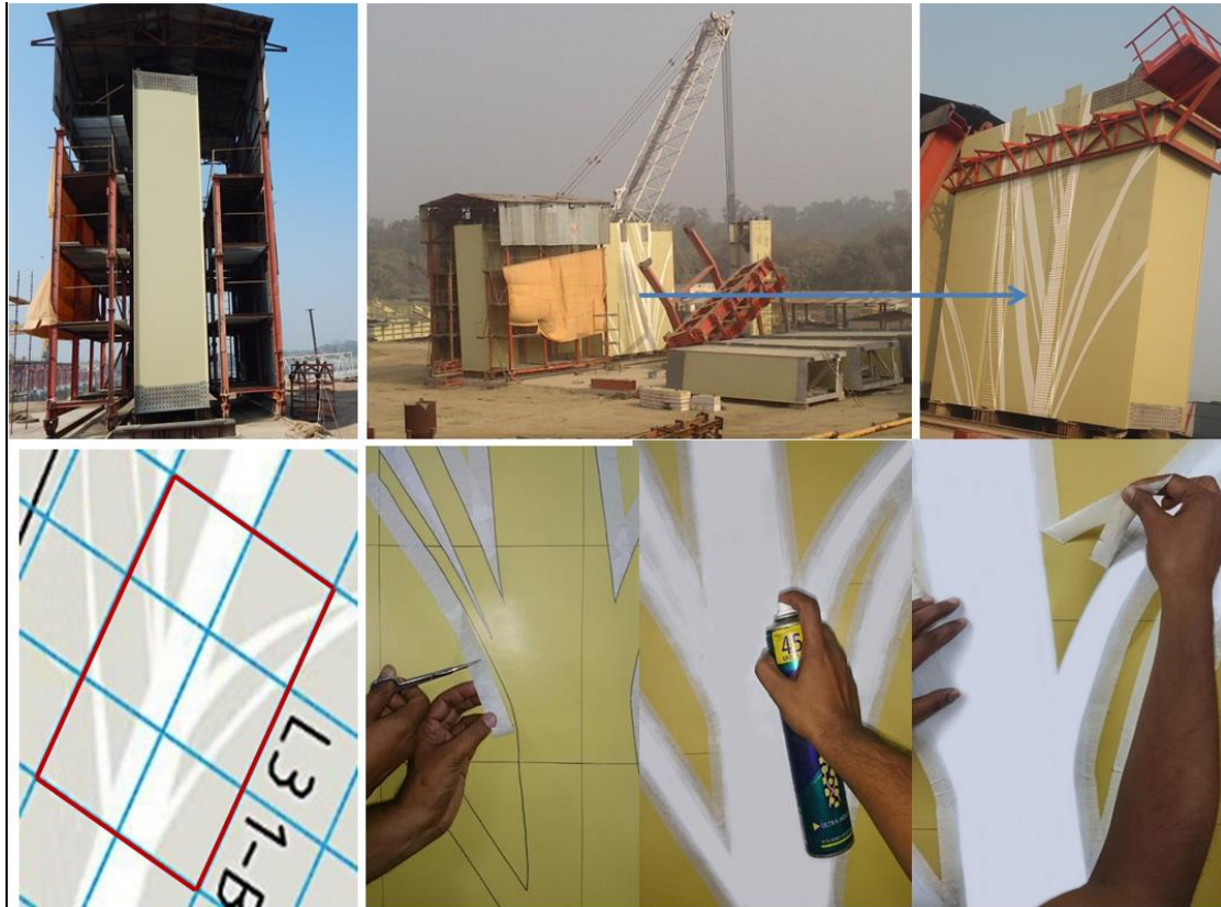
Fig.21. Graphics on pylon during construction
