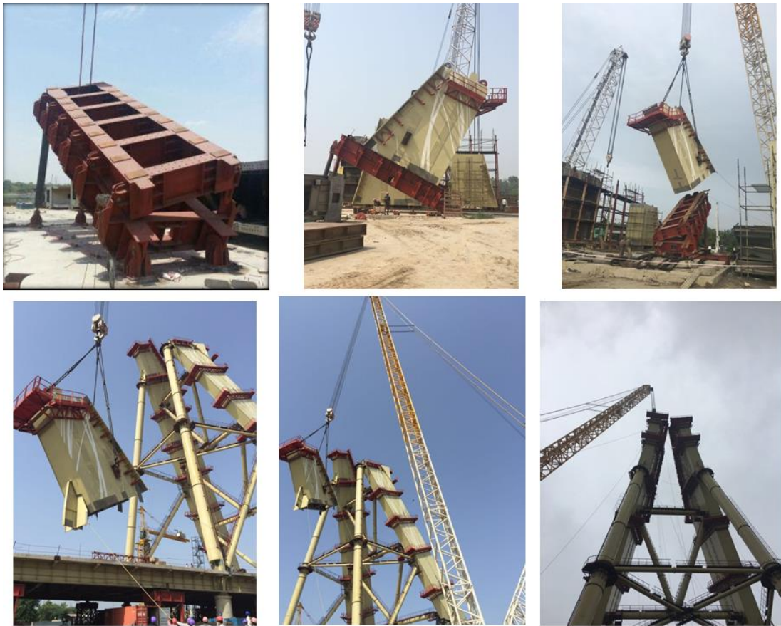
Fig.18 .Specially designed turn table for rigging 3 dimensionally varying pylon segments
