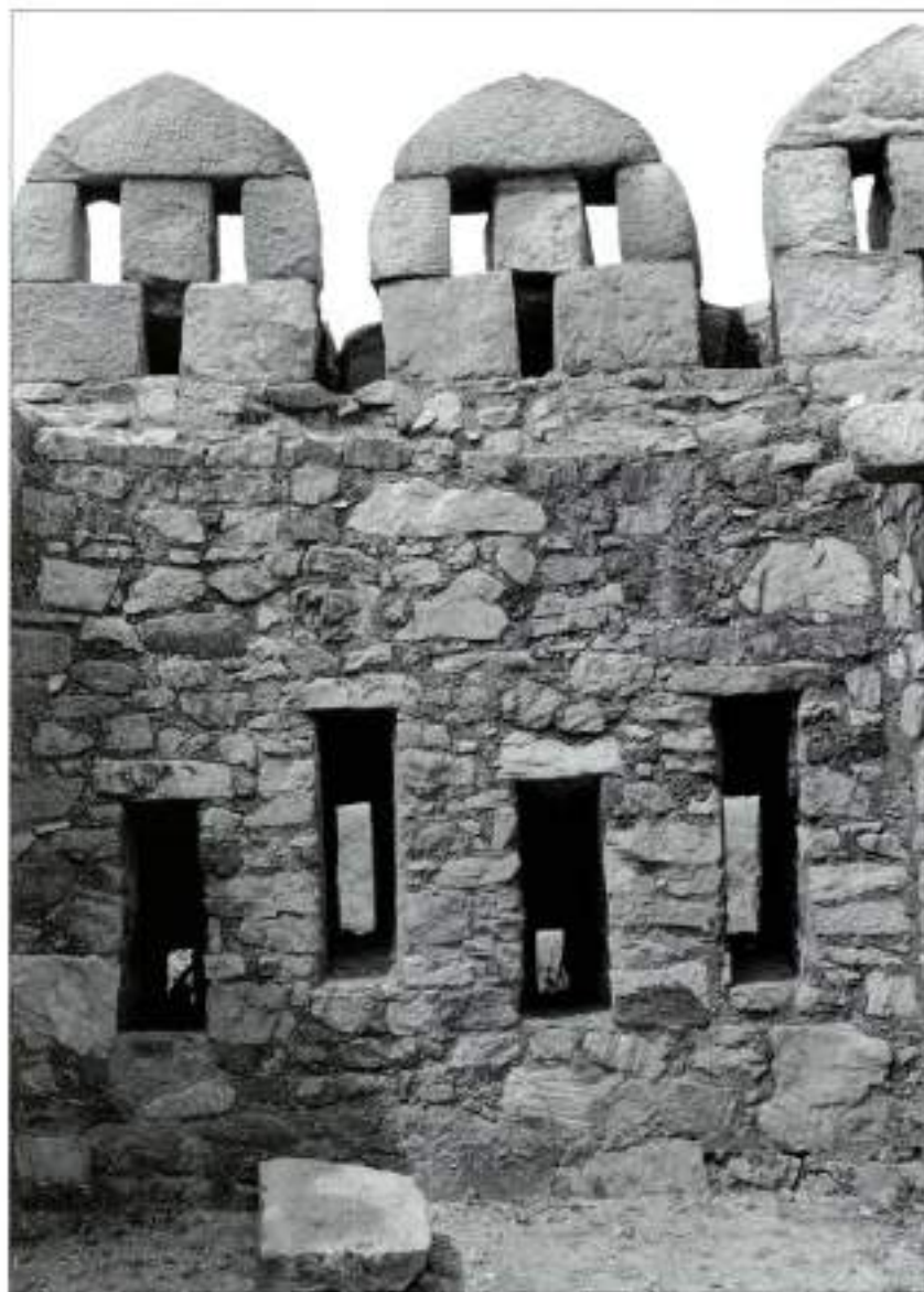
Loopholes and merlons of the barbican tower at the citadel gate in Tughluqabad seen from the inside. The direction of loopholes in the lower row alternates between looking downward and looking ahead. Each merlon in the parapet has three loopholes; the upper two are directed straight out and the lower one downward.
