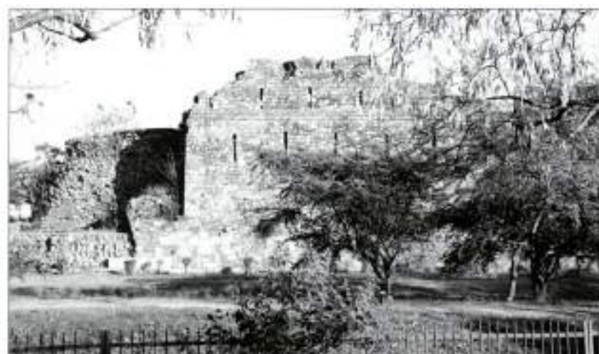
A fragment of the wall of Siri or the second city of Delhi. There were two mural galleries matching the two rows of loopholes in the photograph. The parapet does not survive, but it probably included two more tiers of fire, one in merlons and crenels, and the other through the loopholes directed downward from the parapet.
