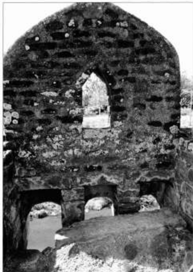
A machicolation in the wall at the Triple Gate in Bidar seen from the inside. Fire could be directed through it right ahead and sideward, as well as down at the ditch. A rectangular loophole with a triangular upper part was designed for handguns. Such loopholes, along with rectangular ones with a rounded upper part, as well as strictly rectangular ones, can be seen in different sections of the walls at Bidar.
