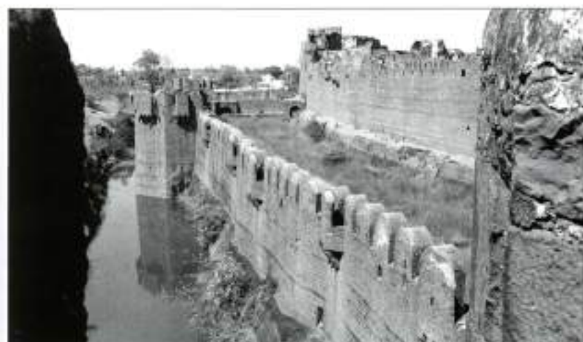
A view, through a crenel, of the walls of Bidar in the neighbourhood of the Triple Gate. Projecting far beyond the wall level, the towers allowed effective flanking fire and command of the entire length of the moat. This was further assisted by box machicolations, which often looked like a merlon projecting beyond the wall line.
