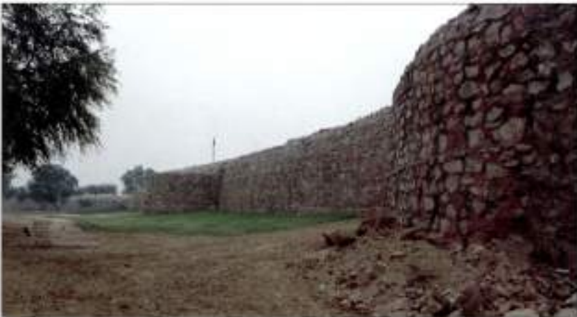
A wall of Qila Rai Pithora or the first city of Delhi, built c. 1180. Laid entirely of rubble, the walls are 5–6m thick in places.
