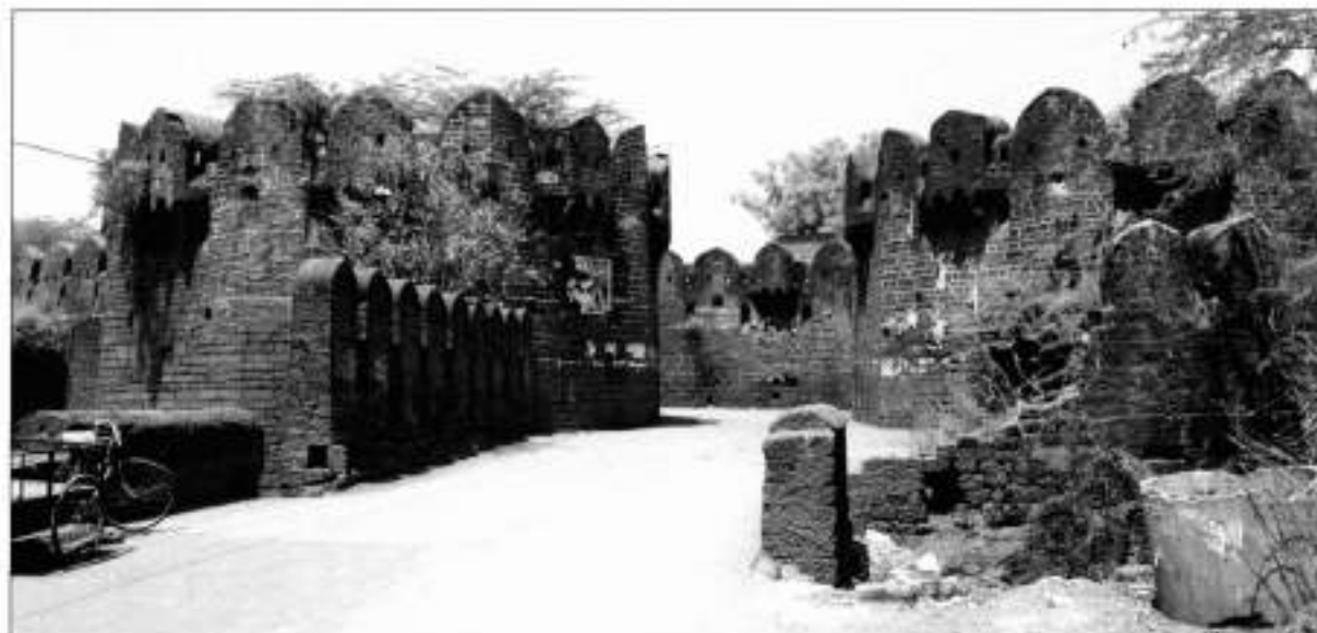
The Fateh Gate – the principal entrance into the lower town of Bidar. The gate was reached by a winding passage flanked at the entrance by two formidable octagonal towers with box machicolations. There also used to be a drawbridge in front of these towers.
