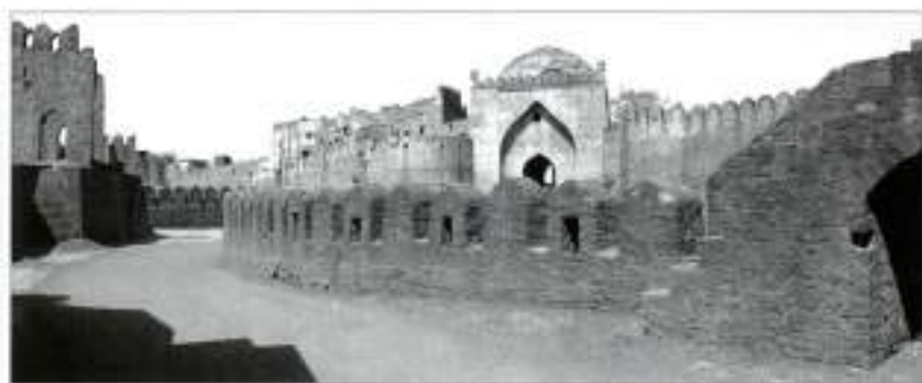
The fortified passage to the Gumbad Gate in Bidar, the third (internal) gate of the Triple Gate dividing the upper town from the lower one. The Gumbad Gate has a domed roof; the gateway widens inside the gatehouse. There are eight arches here, only two of which are for passing through, the rest being 'blind'. This square gatehouse, with a dome and an arched thoroughfare, has all the characteristic features of Muslim architecture.
