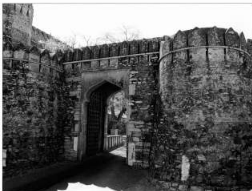
The fifth gate (Jorla Poi) of the western gate complex in Chittorgarh. It is the only gate of the complex obviously rebuilt by Muslims. Muslim influence is particularly evident in the pointed arch. In all the other gates the heads of the passages are constructed with flat lintels and corbels, which is characteristic of Hindu architecture.
