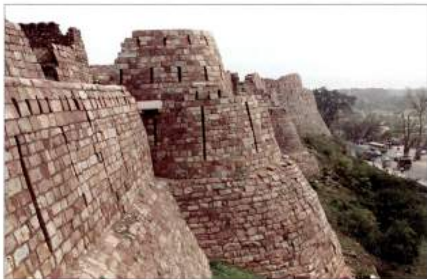
RIGHT The walls of the citadel of Tughluqabad. The walls and towers are reinforced with a solid talus. Two rows of loopholes can be seen on the external and internal walls; another tier of fire was provided by merlons with loopholes, only a few of which survive.
