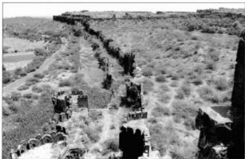
The fortifications of Bidar in the north-west part of the upper town, viewed from the Delhi Gate. Here, the fortifications consist of a double wall and ditch. The citadel on the hill is visible in the distance.
