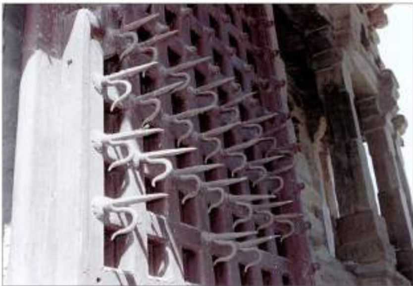
A comparatively rare type of anti-elephant spike with hooks can be seen on this gate of Kumbhalgarh. The spikes only cover a small part of the gate on a level with an elephant's forehead.
