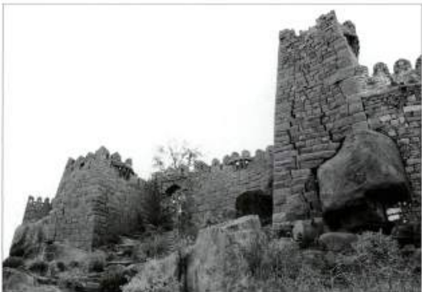
Citadel walls in Golconda. Faced with solid stone blocks free of mortar, these walls are skilfully attached to the huge stone clods of the rock. Two box machicolations, each lying on three corbels, can be seen near the gate.
