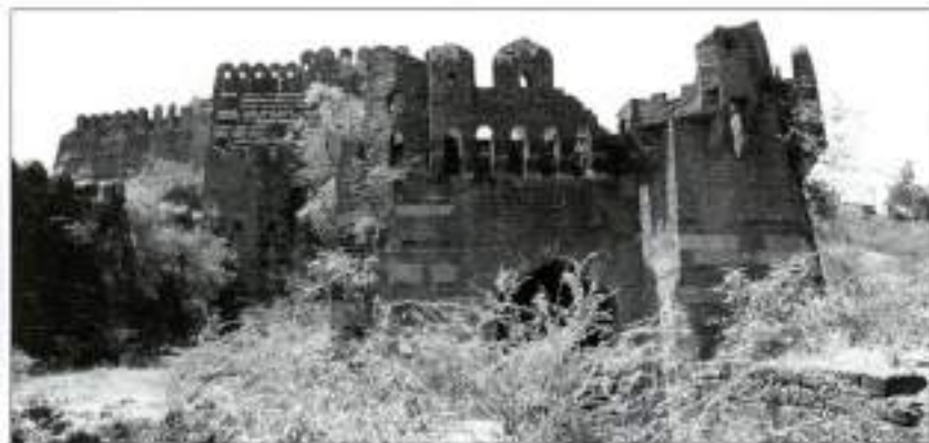
The Delhi Gate in Bidar. The external gate sits in the barbican. The gate is protected with box machicolations from above and one side. In order to get from the external to the internal gate one has to go through the barbican and turn left at 90 degrees.
