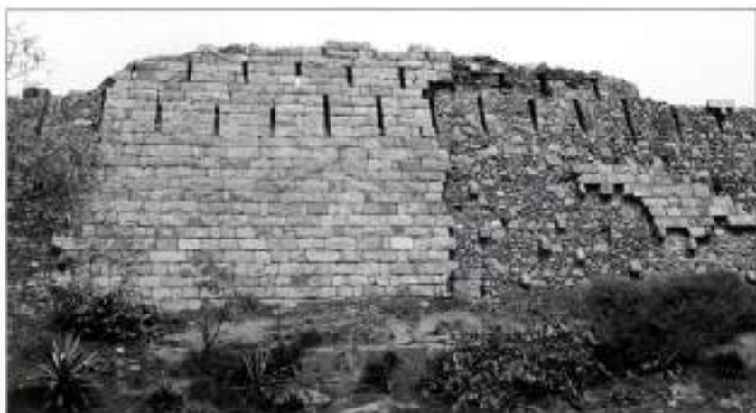
The dilapidated walls of Tughluqabad. The facing has fallen down in places, uncovering a rubble core.
