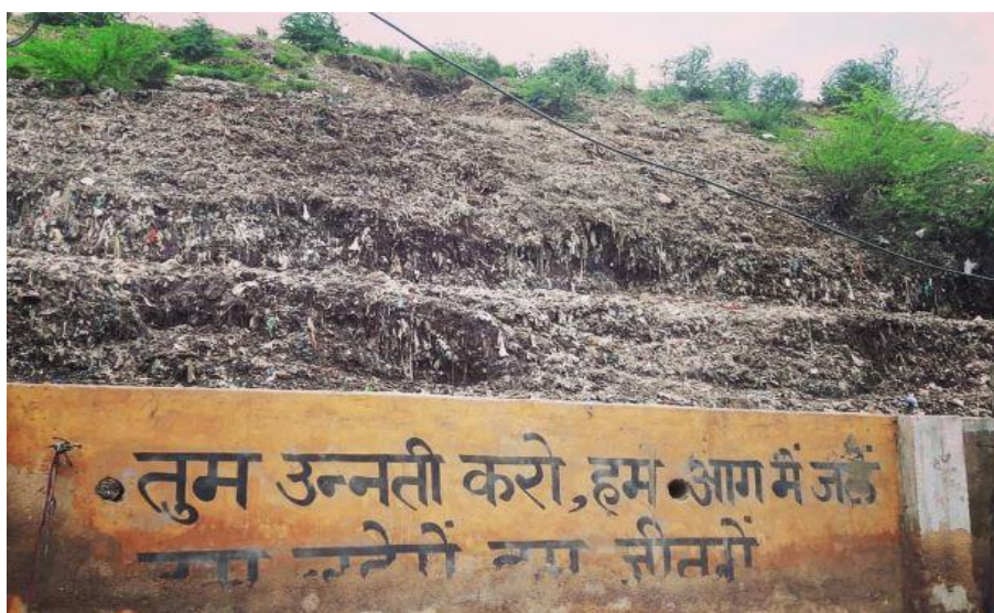
Figure 5.3: Graffiti on the wall of the landfill.
