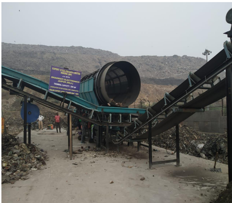
Figure 4.1: The photograph depicts a newly installed trommel machine in front of the Bhalswa landfill. Source: Photograph clicked by the author.
