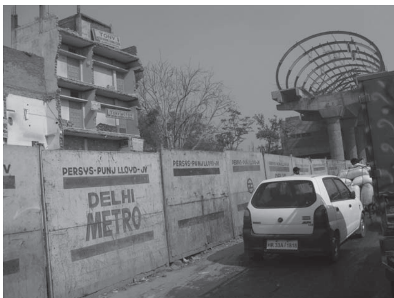
Figure 8.2 Metro construction, west Delhi. Photo by Melissa Butcher
