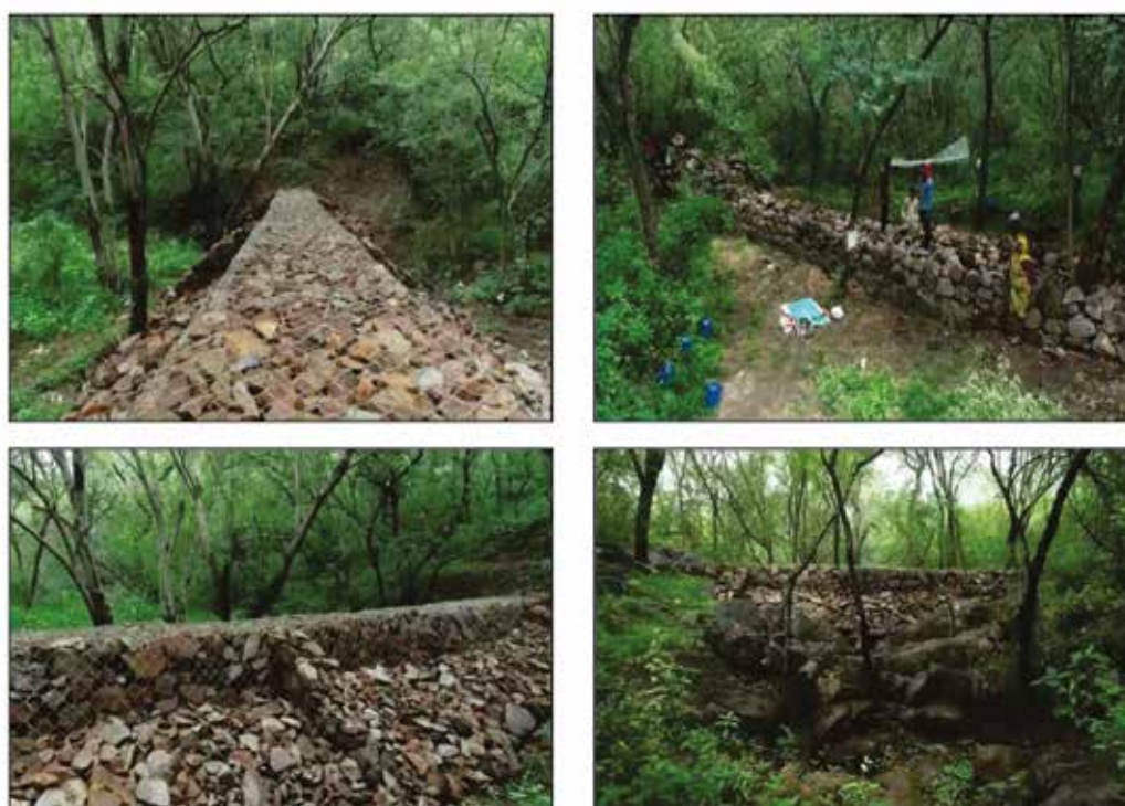
Photographs of Checkdams constructed in Southern Ridge
