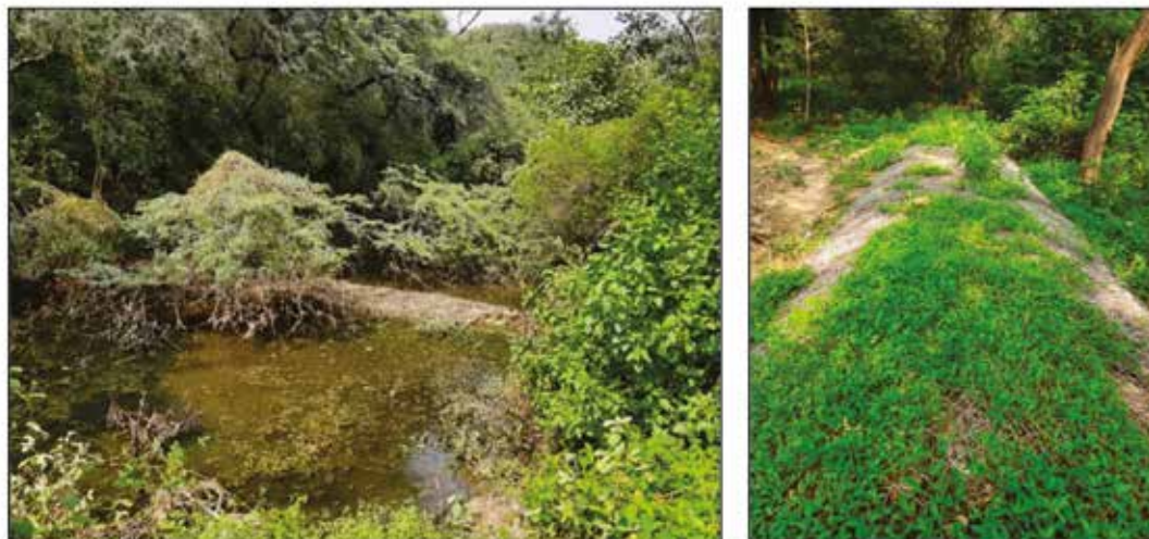
Photographs of Checkdams constructed in Central Ridge
