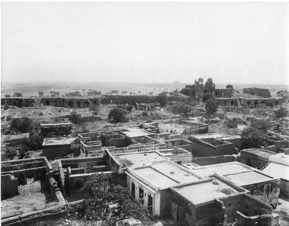
FIG. 4.8. "View Before Demolition of Modern Houses in Baburpura" (P.16063.HRG, MAA, University of Cambridge).
