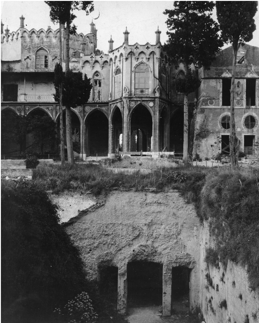
Plate 9 Esther Boise van Deman (1862–1937), Villa Mills on top of the Domus Augustana , 1907. Photographed at the time of its demolition.
