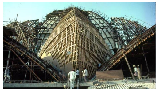
Fig: 11. Formwork
