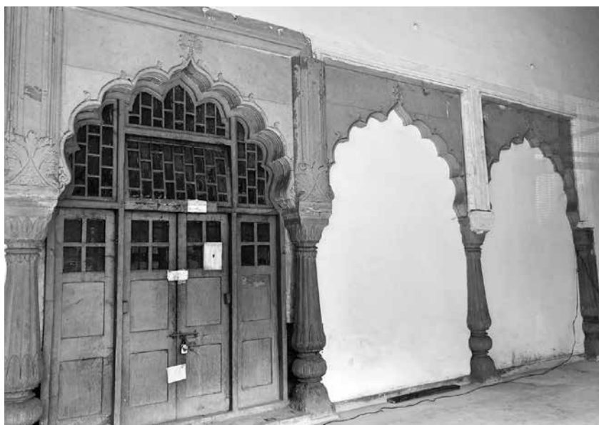
Fig. 12 Delhi Residency, ongoing conservation work on the façade of Ochterlony's 'ball room' with the Mughal era layer conserved Author, 2020
