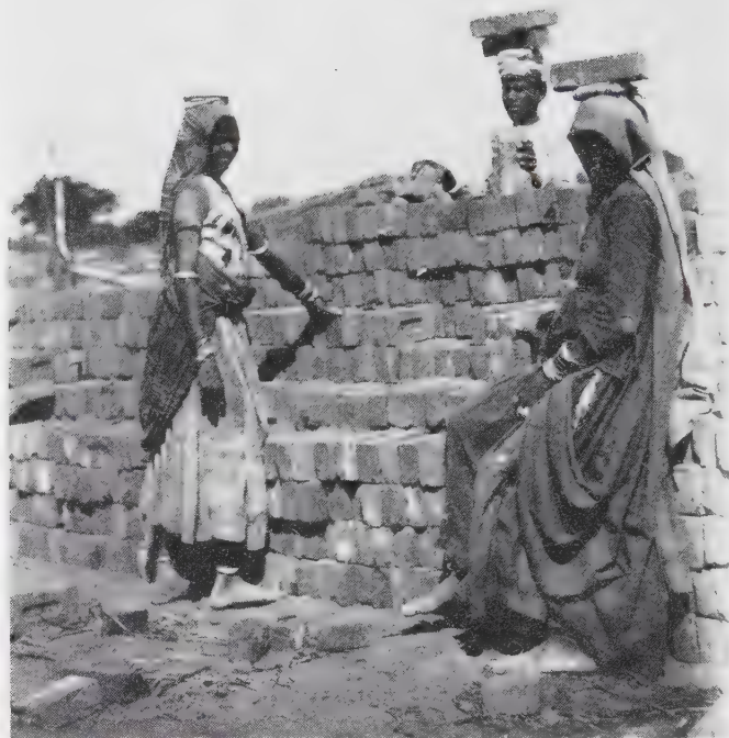
46. Coolies loading their bricks.
