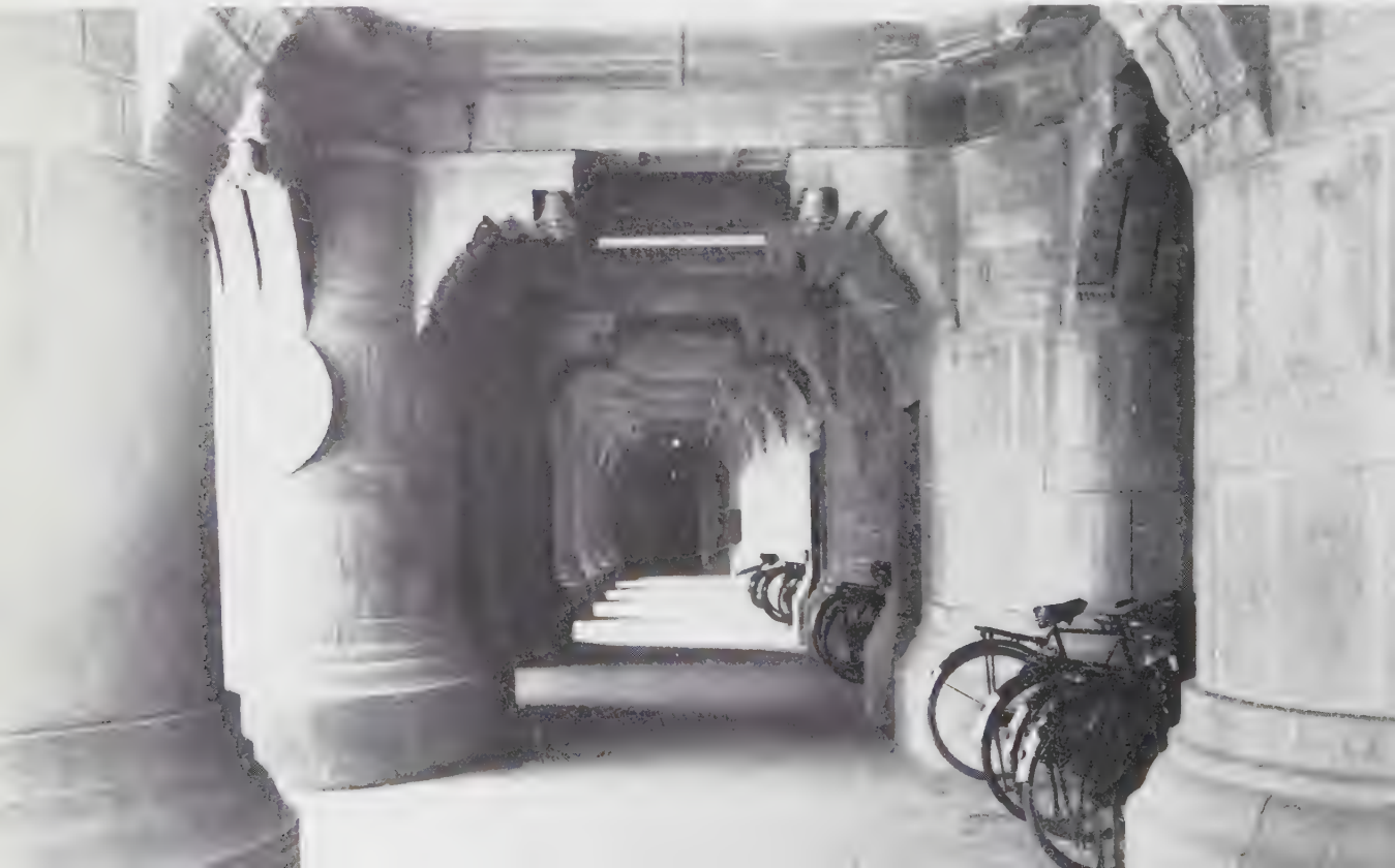
78. Massive kitchen entrance columns, Viceroy's House
