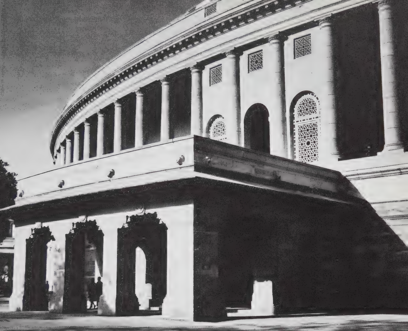
216. Main entrance, Council House.
