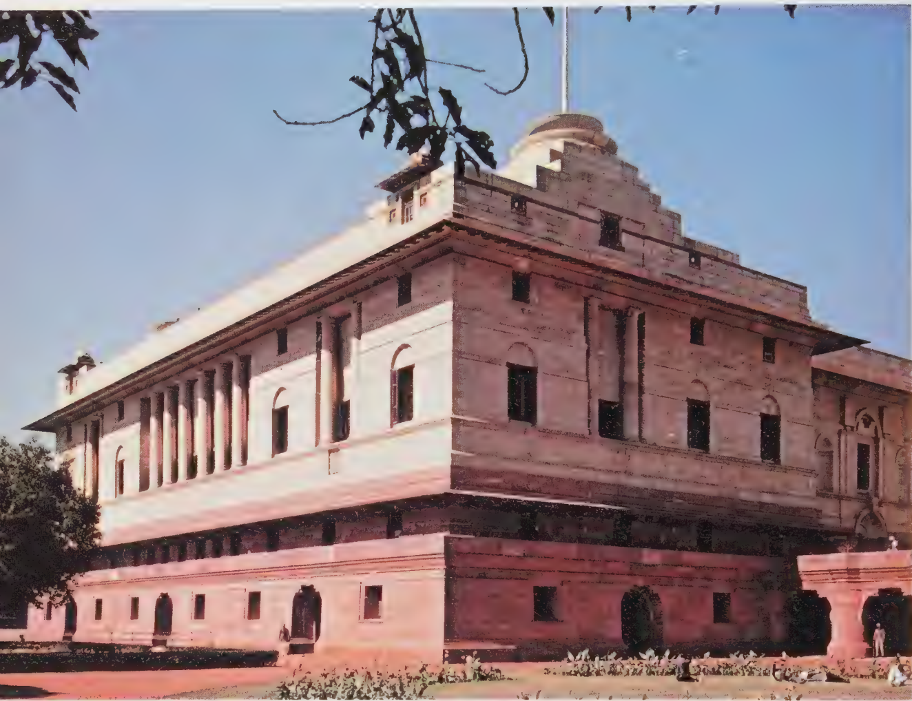
66. The southwest wing of Viceroy's House.
