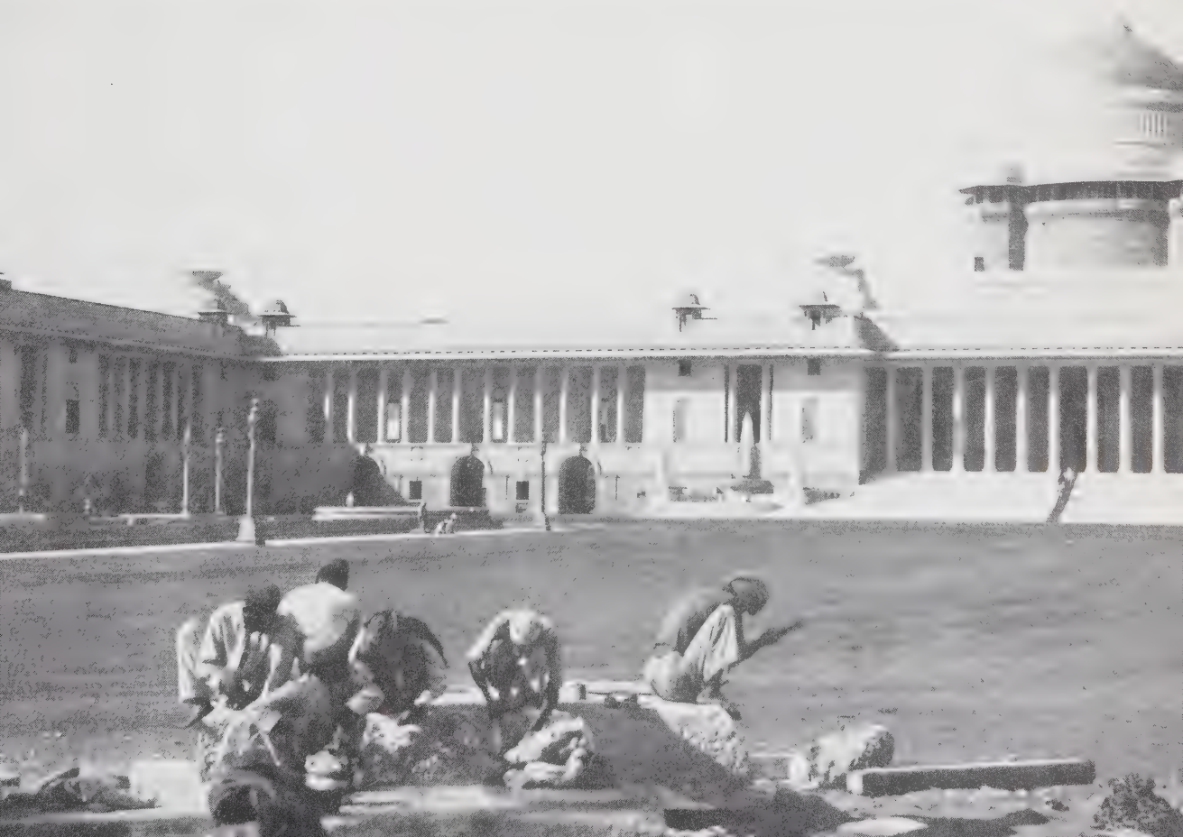
44. Stonecutters preparing the plinth of the Jaipur Column in the forecourt of Government House.
