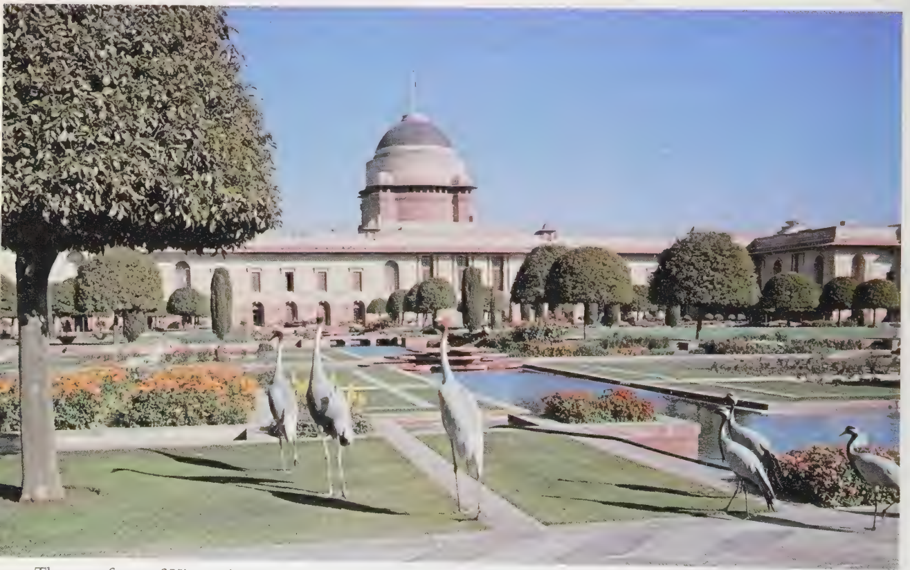
22. The west front of Viceroy's House from the Mughal Garden.
